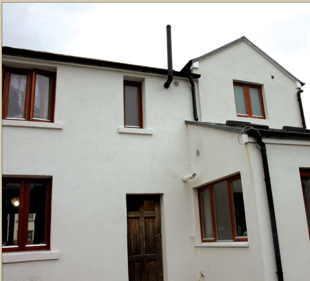
(above) The closed-panel timber frame extension houses a new en suite bedroom upstairs; (below) to maintain a similar appearance, the same double-glazed windows were installed in the two-storey extension, seen here at right, as were previously fitted in the original house; (p49, top) cellulose insulation was installed in the original attic to an average depth of 400mm, while (bottom) a 90 per cent efficient Ravenheat modulating condensing gas combi boiler was also installed
